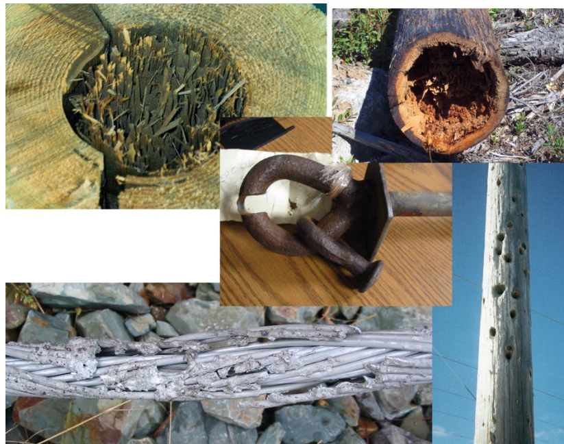
Figure 2: Sample Wood Pole Inspection Results
