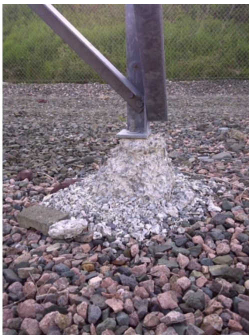
Figure 14: Structure L01L37-1 Western Avalon Terminal Station
