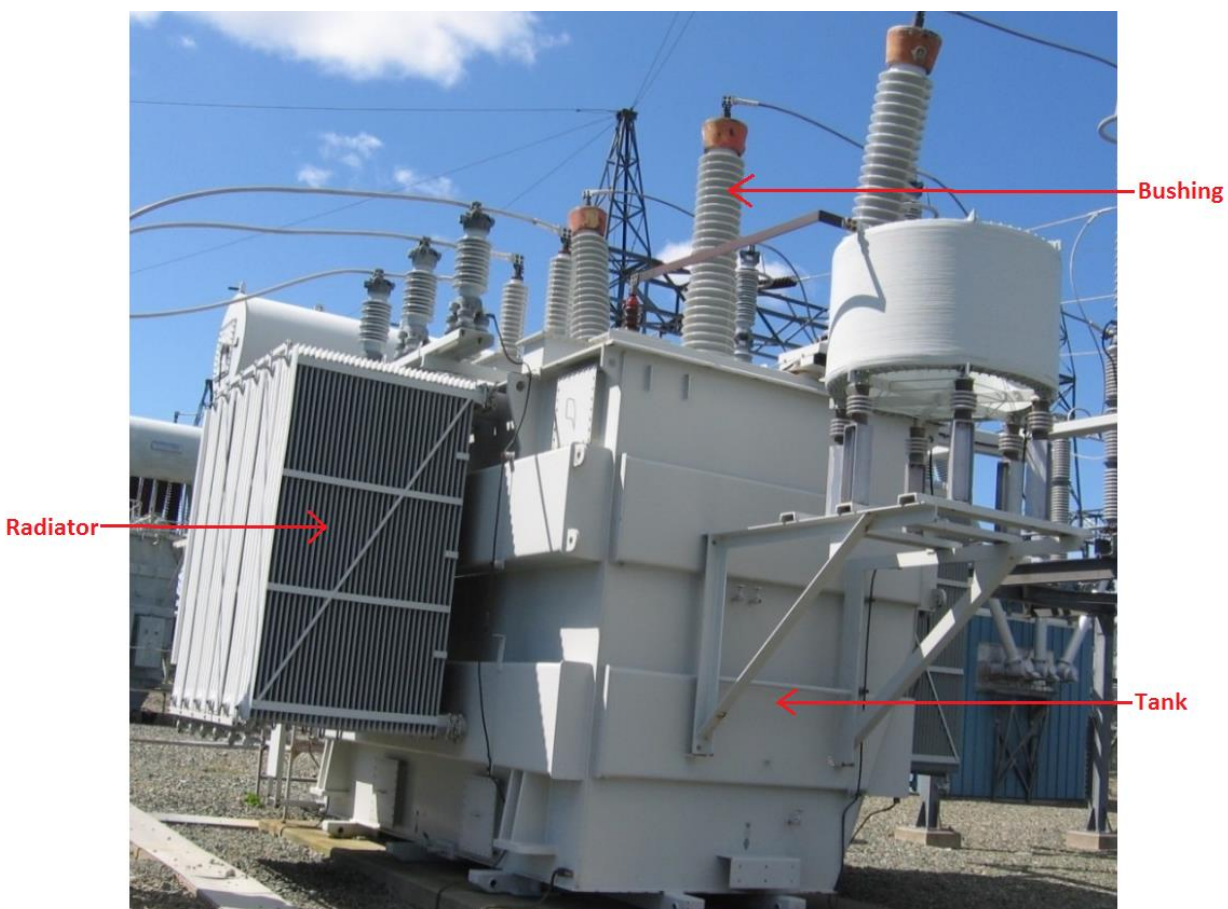
Figure 8: Power Transformer
