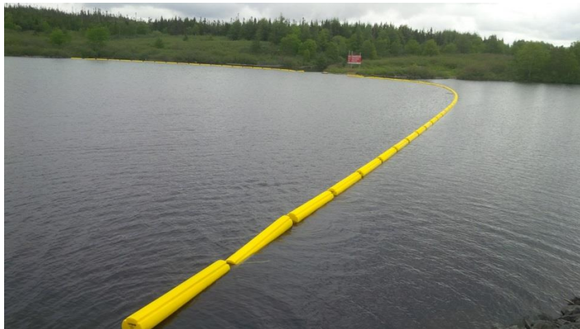
Figure 9: Safety Boom and Signage
