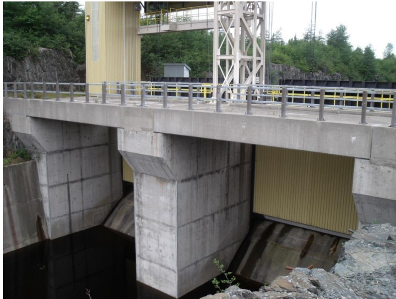
Figure 5: West Salmon Spillway Control Structure
