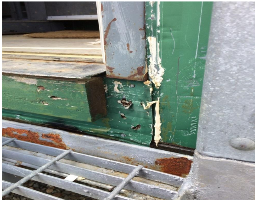
Figure 7: Gull Pond Hill – Exterior Door
