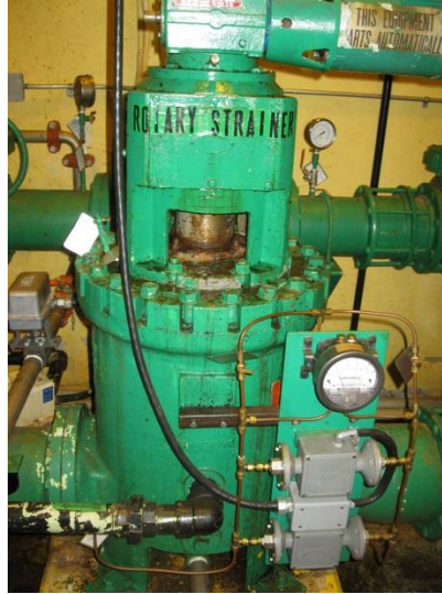
Figure 16: Rotary Strainer
