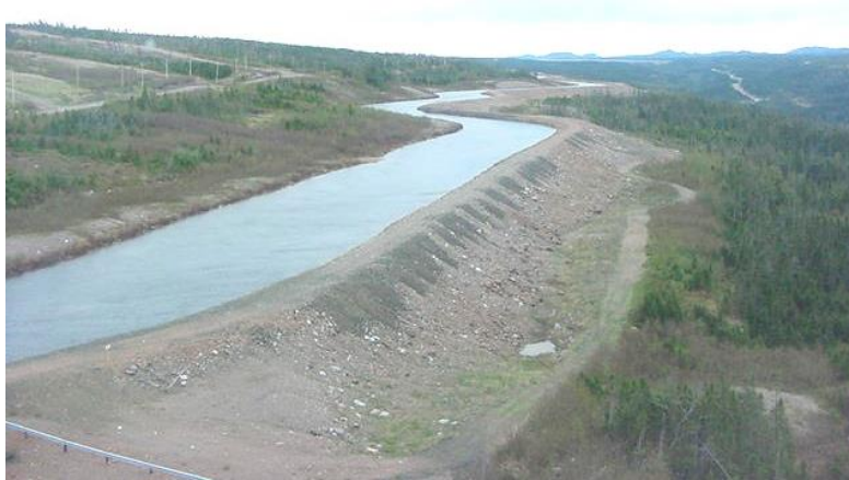
Figure 8: Hinds Lake Power Canal
