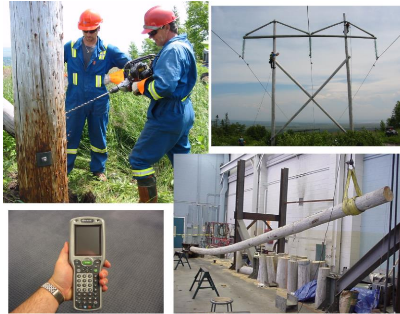
Figure 1: WPLM Inspection Techniques, Clockwise from Bottom Left: 1) Typical Field Data Collector; 2) Cavity Measuring; 3) Climbing Inspection; 4) Destructive Testing at MUN
