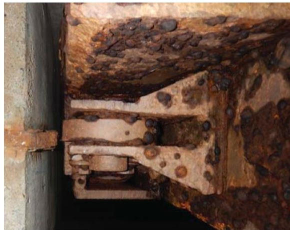
Figure 9: Seized Side Roller - Ebbegunbaeg
