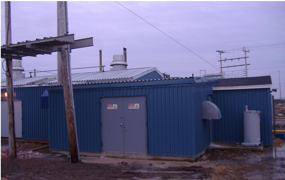
Figure 1: Black Tickle – Diesel Generating Plant
