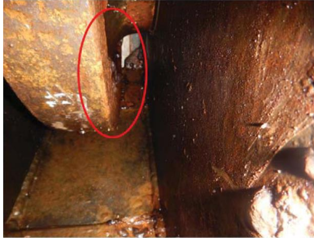
Figure 8: Roller Corrosion - Ebbegunbaeg
