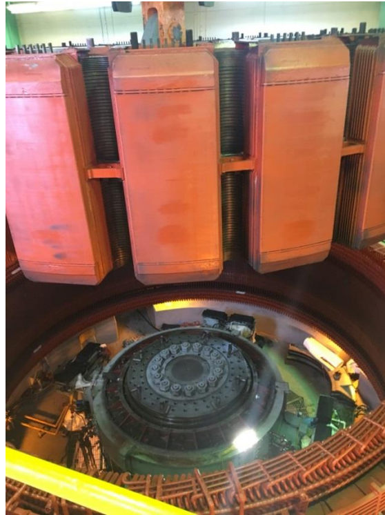
Figure 3: Dismantled Generator
