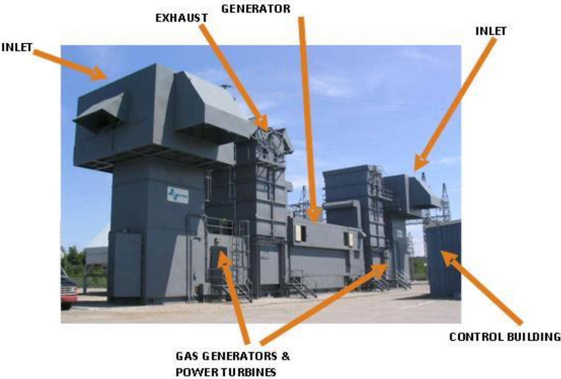
Figure 1: Stephenville Gas Turbine Plant
